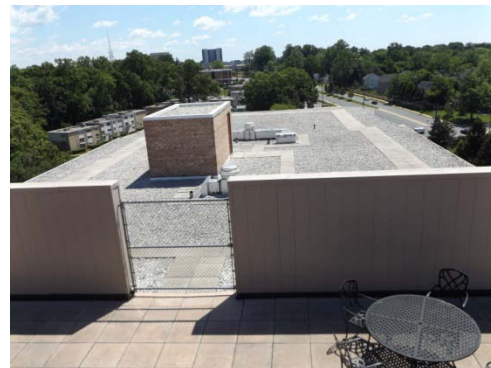
Photo 9 - Roof section being replaced
