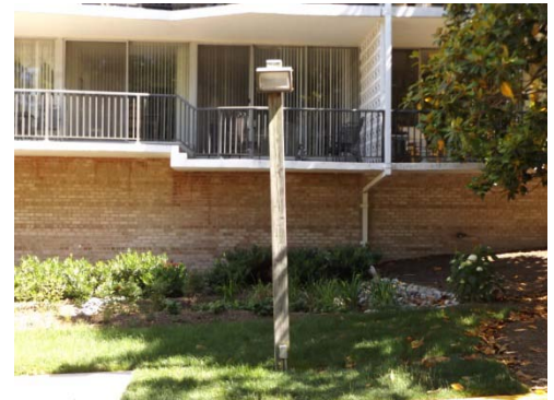
Photo 4 - Site light fixture
