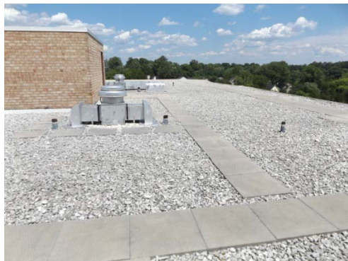
Photo 8 - Inverted roof
