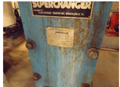
Photo 20 - Heat exchanger
