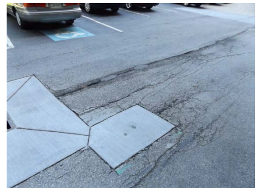
Photo 2 - Deteriorated asphalt
