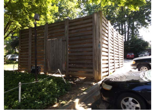
Photo 3 - Cooling tower enclosure
