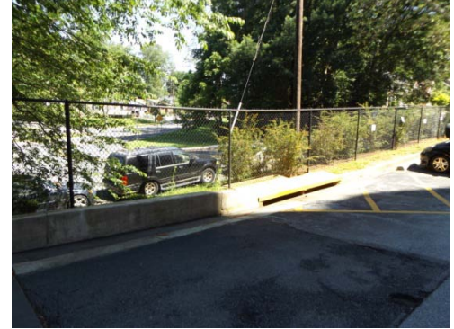
Photo 6 - Retaining wall fence
