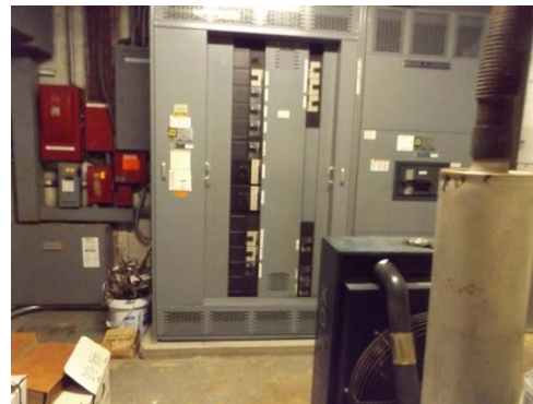
Photo 22 - Primary switchgear
